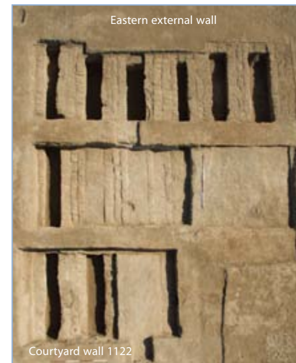
Plan and drone photo (SE at top) of the six sub-floor vaults in the Public Building.
